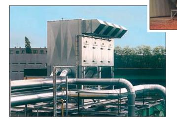
Filter system for 240,000 m³/h for window factory in Scotland with silo system for storage of chips before combustion.
