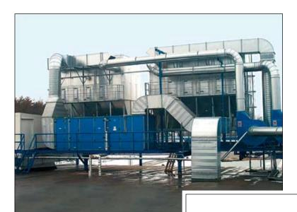
Modular constructed filter systems type AKF-WDHK and AMX are intended for large volumes of air and chips. The filters are very reliable and flexible by rebuilding and extension, at the same time they are cleaned automatically during operation and can run in 24 hours operation all the year round under all operating conditions.
