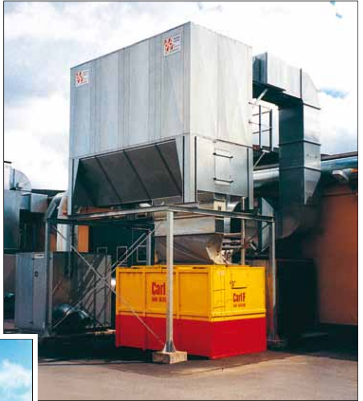
Rotary valve filter on standard container stand for existing containers.
