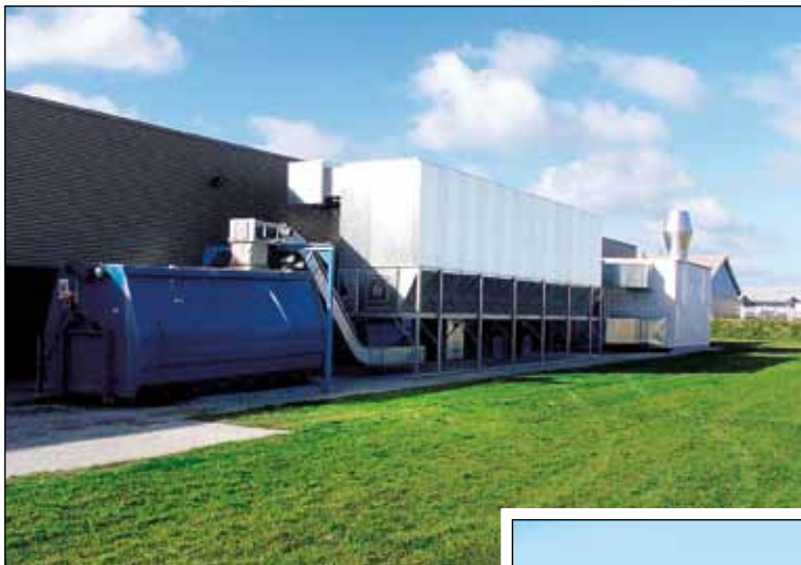
Filter system type AKF-DHLK with cross heat exchanger for the return air to the factory and with chip conveyor for transportation of chips to container. Supplied to Danish furniture joinery.
